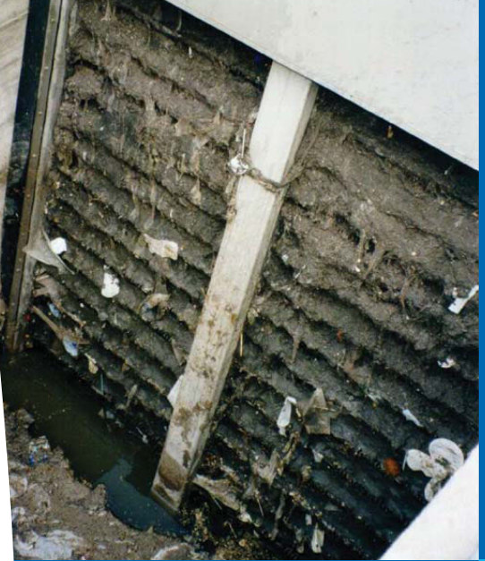
Figure No. 3 Double Wide Installation
